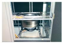
The existing AHUs are fitted with two fans each. Retrofitting those units with GreenTech EC centrifugal fans (RadiPac) made it possible to achieve energy savings in the units of up to 70%. What is more, thanks to the EC fans, the systems can now also be closed-loop controlled to actual demand.
