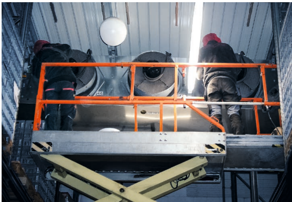
Out with the old AC fans: The retrofit with modern EC fans aims to help Emmi reduce its own emissions (Scope 1 and 2) by 60 percent by 2027.
